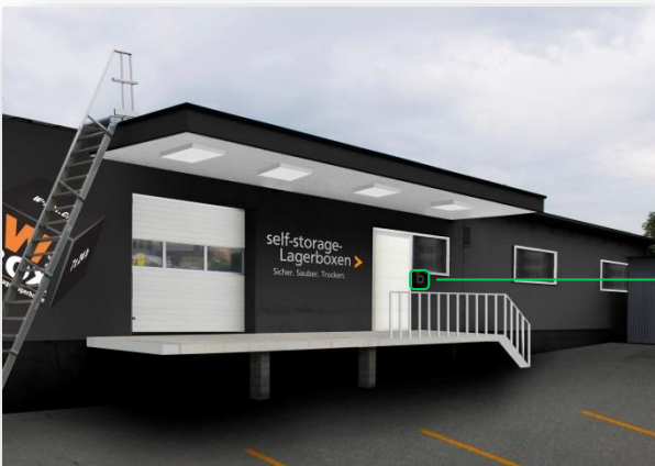
Please hold your keycard to the KABA-sensor on the right side of the entrance door...
