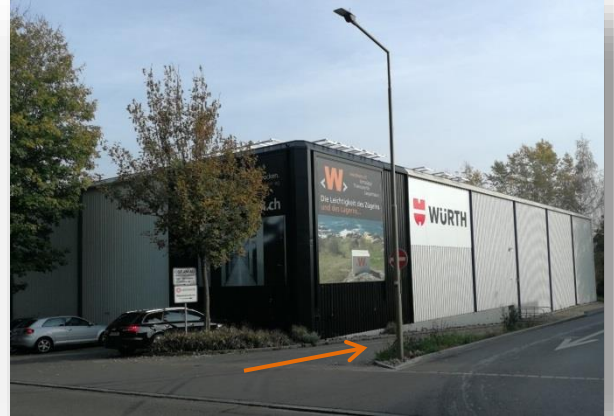
Access is only allowed from this side. Here you will find the entrance to the stairs.
